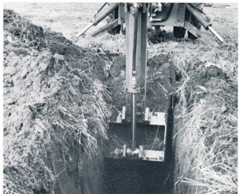
Bucket digs 6 feet and 4 inches deep.
