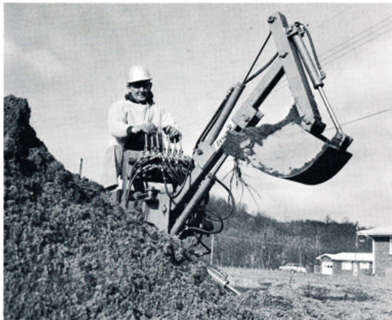
Dig deep, dig straight at low cost.
