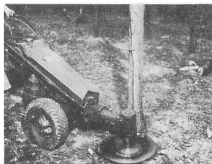
CLEAR LAND, CUT TIMBER
