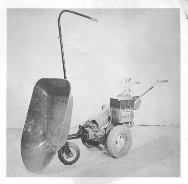
Just raise the Handle to dump. The Handle is designed to be always within easy reach of the operator.
