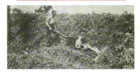
The GRAVELY Model D is not just a single purpose machine. Besides being the best power narrow row cultivator, the GRAVELY, when equipped with the Sickle Mower attachment, will cut grass, weeds and brush as high as your head and as thick as your thumb.
